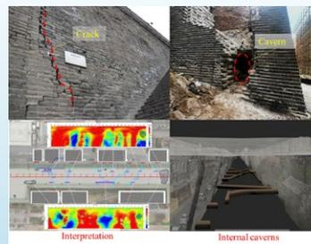
↑ Xi'an City Wall Damage and Geophysical Exploration
